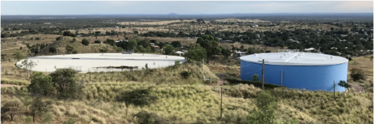
Above: Water tanks on Towers Hill.
