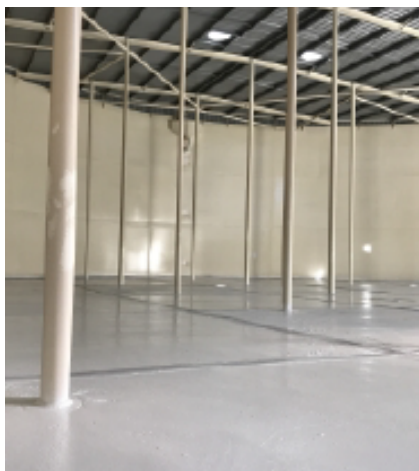
Above: Inside water tank built 1985
