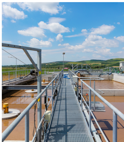
Above: Example of Water Treatment Plant
