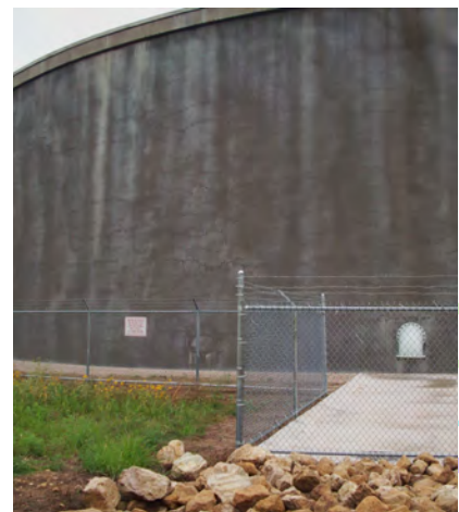
Above: Example of water reservoir
