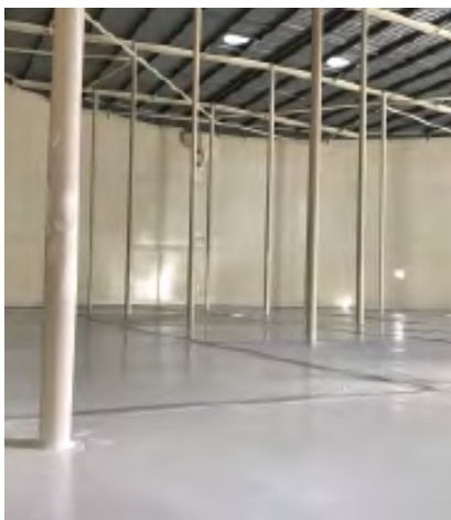
Above: Inside water tank built 1985
