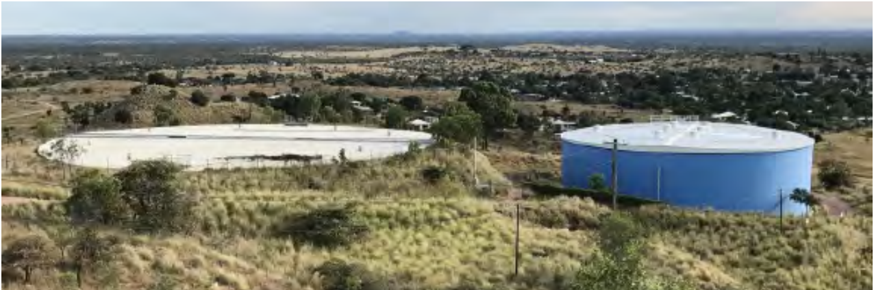
Above: Water tanks on Towers Hill.
