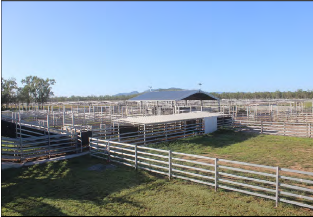
Figure 1: Example of existing infrastructure that will be used
