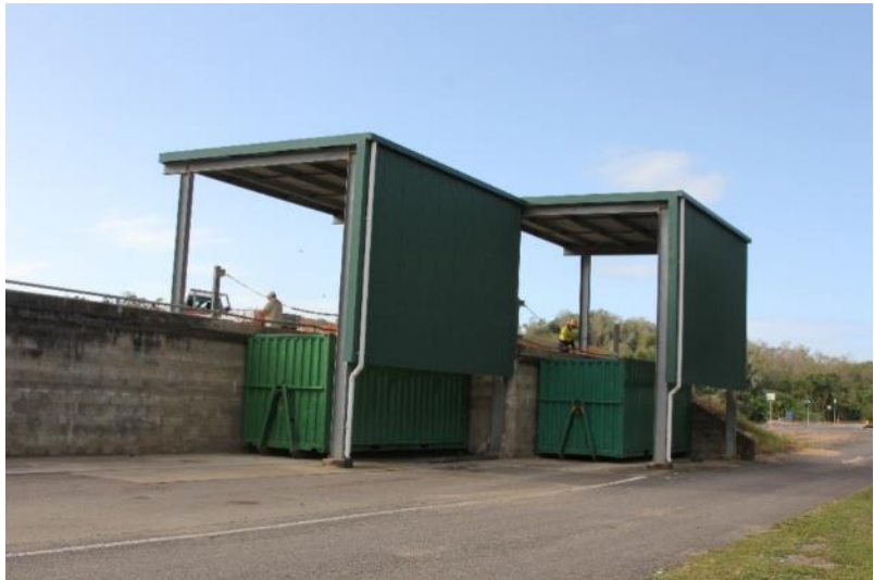
Warrens Hill Resource Recovery Centre, Hinchinbrook
